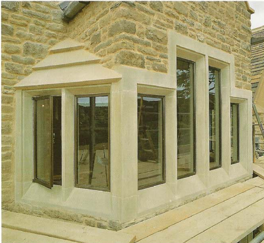
Double glazed, weather stripped bronze window frames provided for a Grade II listed building were manufactured using bronze extrusions and factory patinated prior to delivery.
